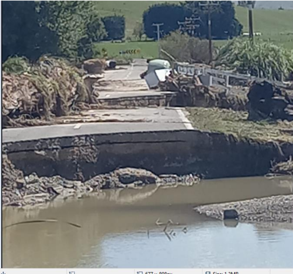
Old Waipawa River Bridge
