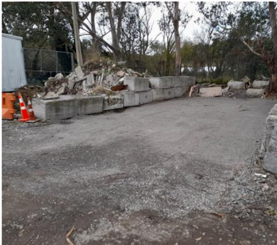
Repairs and resurfacing of green waste bunkers at Waipukurau Transfer Station.
