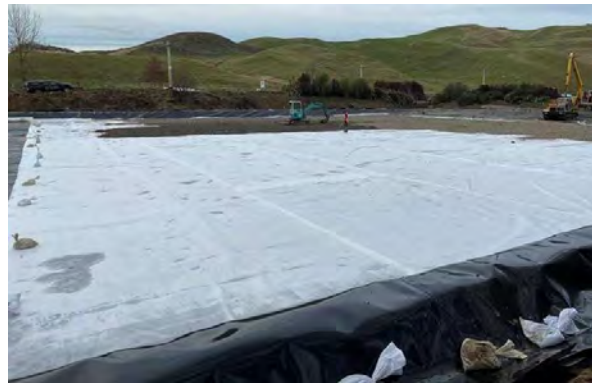
Preparation of the geobag area at Waipawa WWTP for desludging
