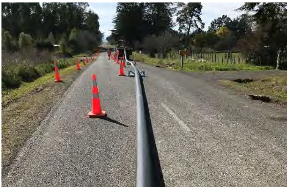
Stage 1 of the Otane to Waipawa Wastewater Pipeline
