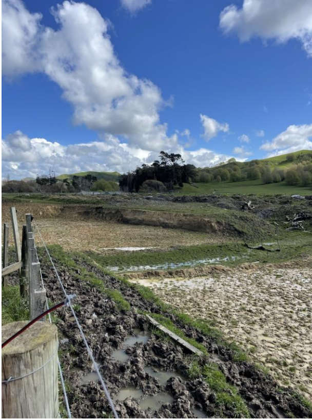
Figure 11: Looking south-west over extensive earthworks and rubbish pile in the location of Lot 15. Source: Kate Hooper, 15 September 2022
