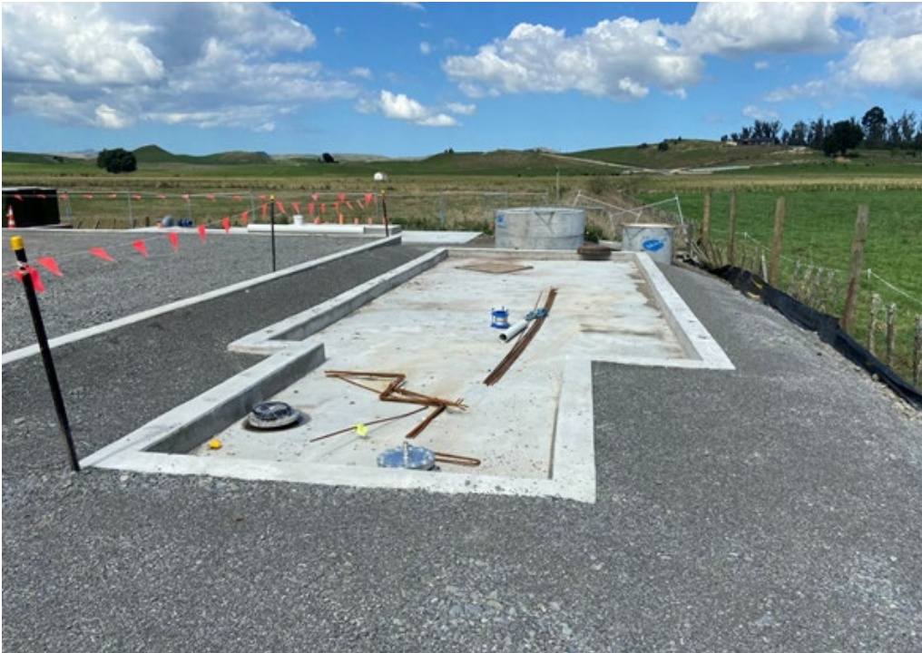
Figure 2: Otane Pump Station – awaiting pumps and pipework
