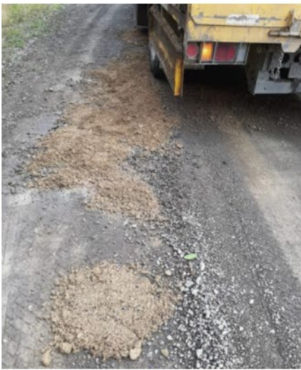
Mill Road- After Photo
