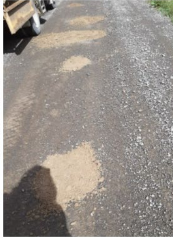
Mill Road- After Photo
