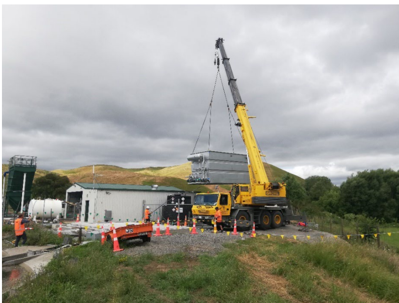
Figure 4: DAF unit craned into place
