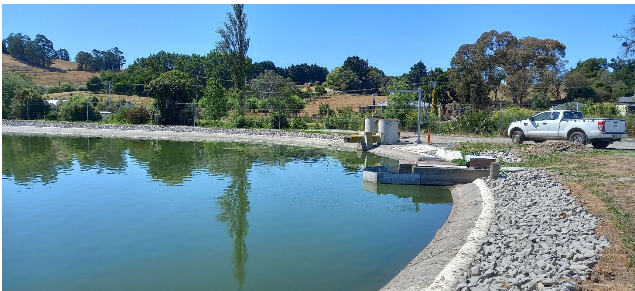
Figure 2: Waveband upgrade/ repairs at Waipukurau WWTP
