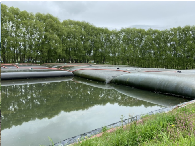
Figure 1: Waipawa desludging - geobags filling
