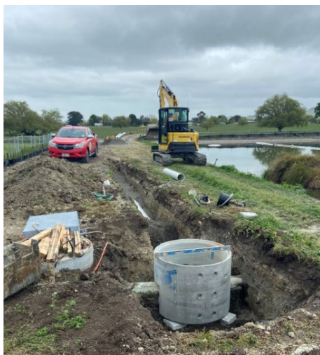
Figure 3: Otāne pump station construction
