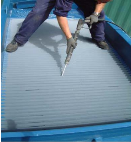
Figure 7 – Illustration of Lamella Plate Cleaning
