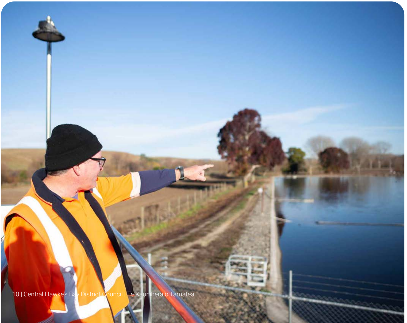
Below: Veolia Waste Water Technician - Ken Sanderson.
